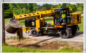
operator Kevin Holy is using an XL 3100 V Gradall to relocate a drainage ditch further from the road for better drainage, and then evenly spread rip-rap the length of the ditch. Without this work, water from a nearby orchard would wash out the ditch.
