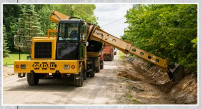
which is not paved and is located in a rural portion of Geauga County, operator Ron Quercioli uses another XL 3100 V Gradall for ditch widening. He places piles of rip-rap periodically to create silt screens and cuts the berms properly to let water run off the road evenly. ❖ "Gradalls
