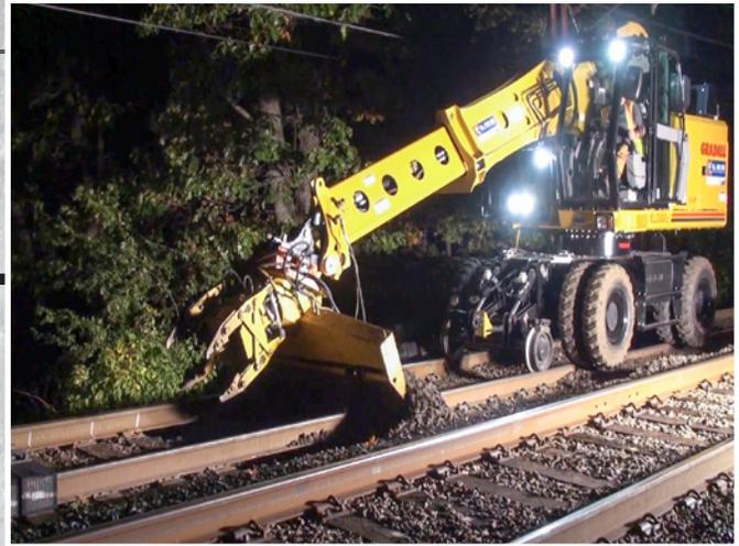
“We chipped out the concrete, poured new concrete slabs and then installed the new rails.” ❖ One Gradall machine, traveling on rails at speeds up to about 15 mph, was used to tow an 8 x 20-foot
